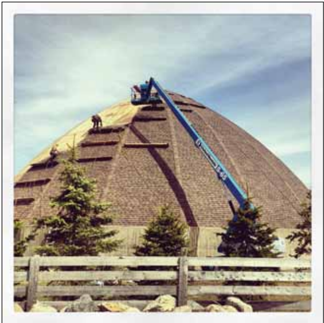
OUT WITH THE OLD, ON WITH THE NEW Creemore photographer MK Lynde captured these great shots of the Simcoe County sand domes just west of town, which have been reclad with new shingles over the past couple of weeks. The photo on the left was taken last week after the old shingles had been stripped off; the one on the right earlier this week as new shingles were being put on.
