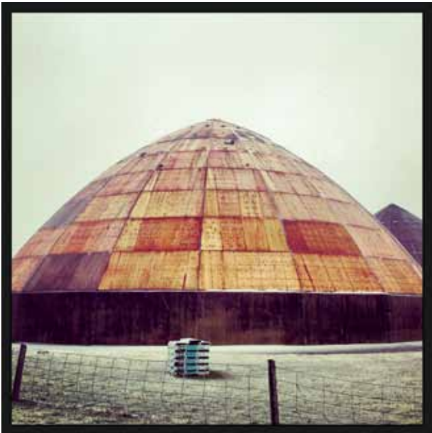
OUT WITH THE OLD, ON WITH THE NEW Creemore photographer MK Lynde captured these great shots of the Simcoe County sand domes just west of town, which have been reclad with new shingles over the past couple of weeks. The photo on the left was taken last week after the old shingles had been stripped off; the one on the right earlier this week as new shingles were being put on.
